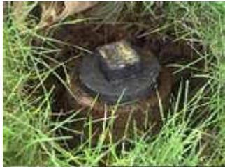
Typical sewer cleanout with properly installed plug.
